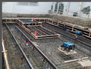
CORE DRILLING & COMMERCIAL SHORING
